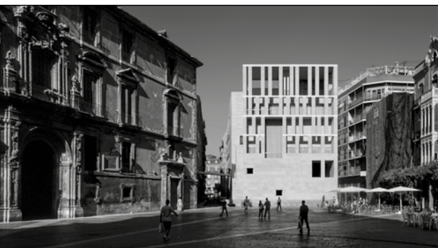
Murcia City Hall extension, 1991-1999 Murcia, Spain
