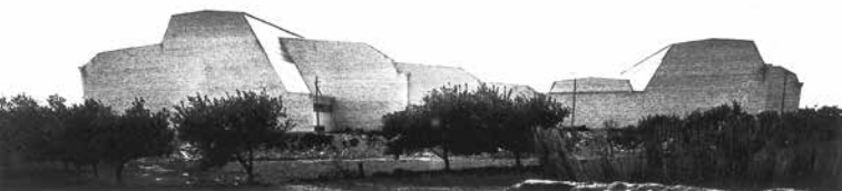
Diestre Factory, 1964 Zaragoza, Spain
