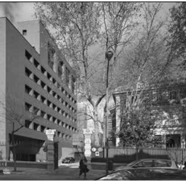
Bankinter headquarters, 1972-1981 with Ramón Bescós Madrid, Spain
